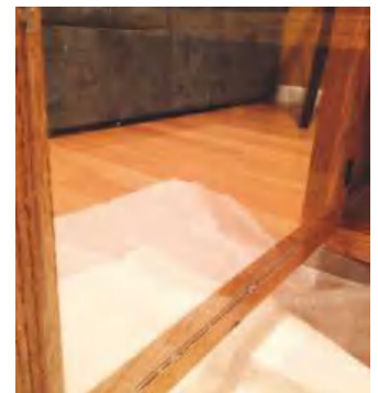
STEP 26. Add mirror tacks for additional holding of the plexiglass, then install the knobs
